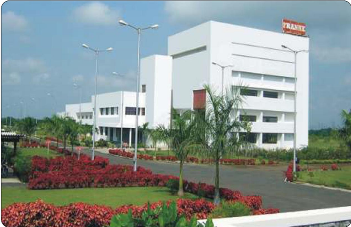
Franke Kitchen Sink Manufacturing facility at Aurangabad, India
